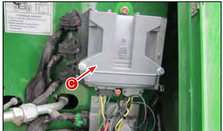
C - Leveling Controller
